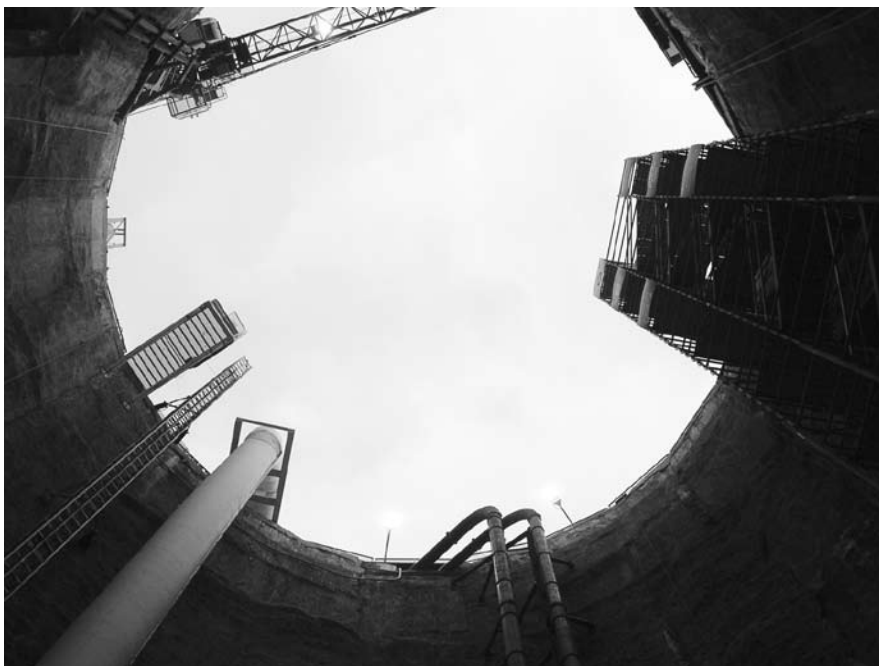
Top: A view of the tunnel straight-a-way on its 6-mile path. Above: A look up from the 115-foot Opera Shaft.
