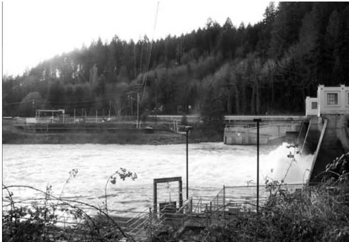
Leaburg Dam on the McKenzie River.
